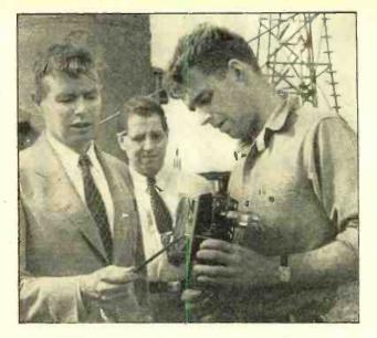
CHECKING THE U.H.F. BALLOON TRANSMITTER Experts of the Weather Station at Blue Hill Observatory making a final check on the ultra-short-wave equipment for the crewless balloon.
