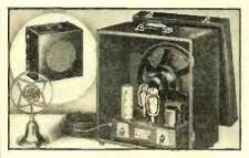
other applications requiring sound equipment of low power. The amplifier employs a type 6F5G tube in the input highgain circuit, a type 6B5 dual-triode tube in the output stage and a type 83 tube serves as the rectifier. Field current is provided for an 11 inch, 2,500 ohm dynamic type speaker. The complete system includes the amplifier, tubes, speakers, a double-button microphone mounted on a banquet stand, and all necessary cables and plugs.
